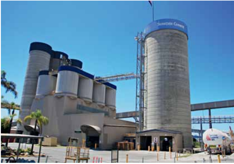
1 Drymix building with storage silos
