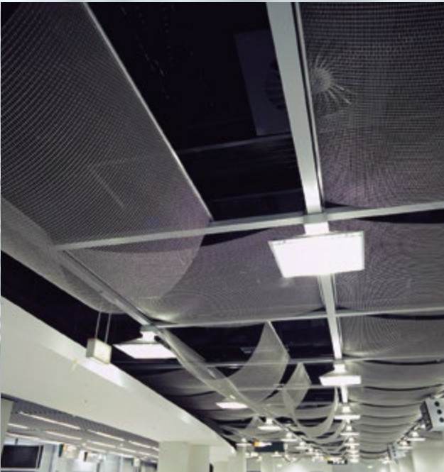
Adjustable mounting system for ceilings with sag.
