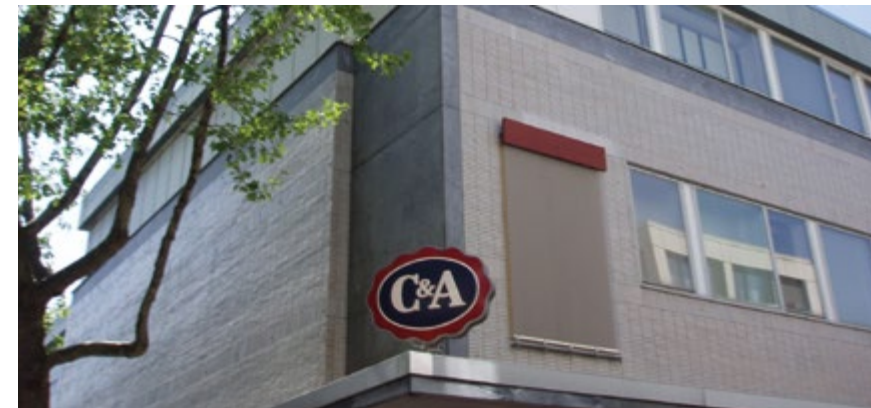
The semi-transparent stainless-steel mesh LARGO-NOVA 2017 encloses the existing building and ensures natural lighting. C&A Eco Store, Mainz, Germany.
