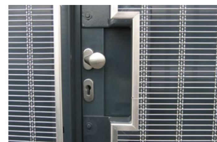
Mesh with edge protection profiles.
