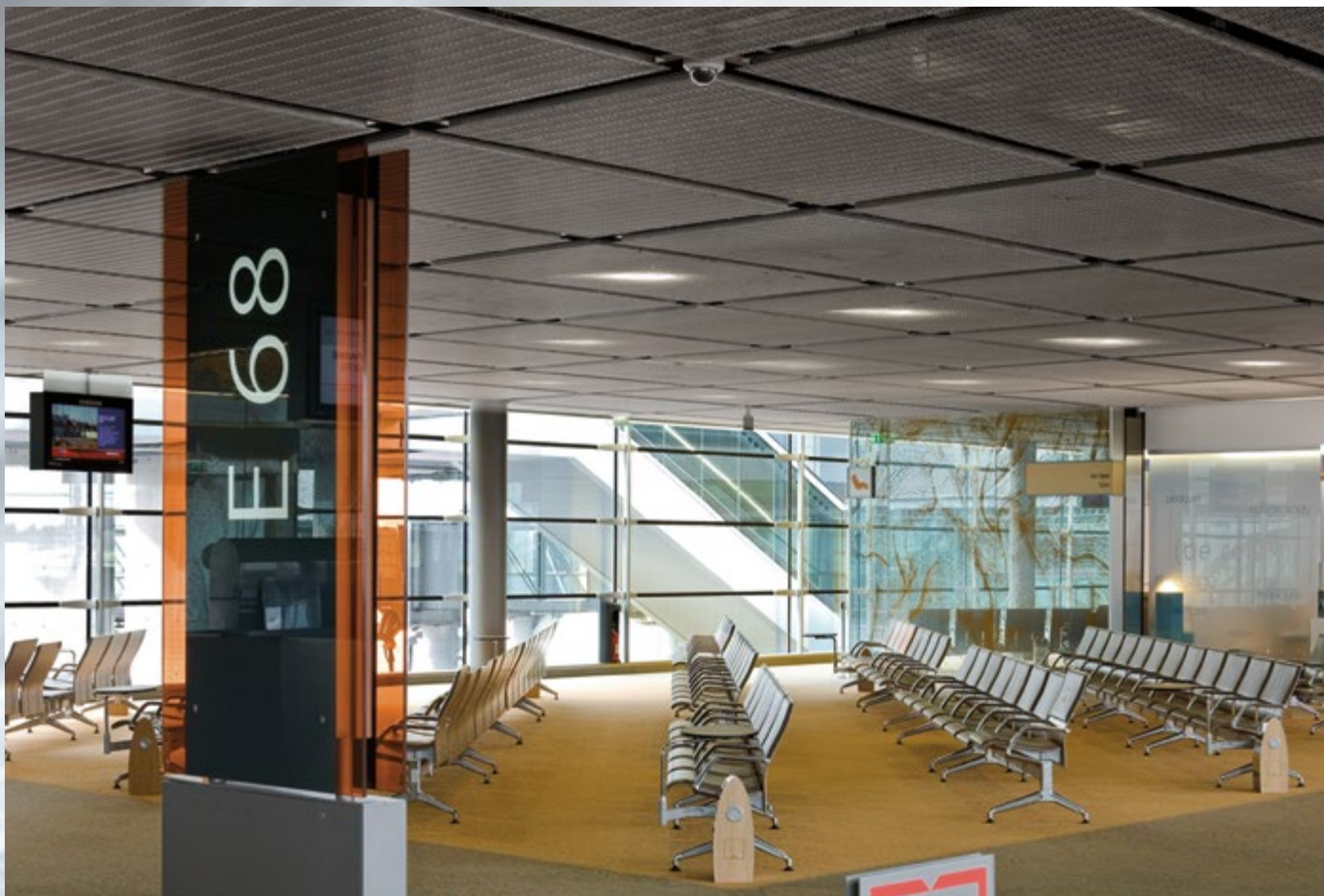
Architectural wire mesh guarantees the optimum operation of ventilation or sprinkler systems. Terminal S3, Roissy Charles de Gaulle Airport, Paris, France, DOGLA-TRIO 1010.
