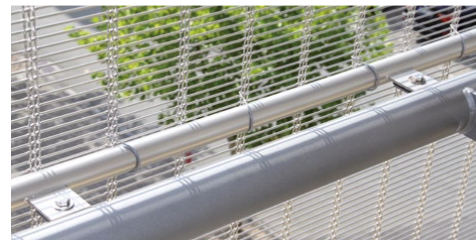
Intermediate mounting: round tube and wire connectors.
