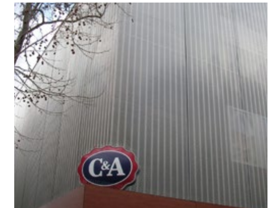
The semi-transparent stainless-steel mesh LARGO-NOVA 2017 encloses the existing building and ensures natural lighting. C&A Eco Store, Mainz, Germany.
